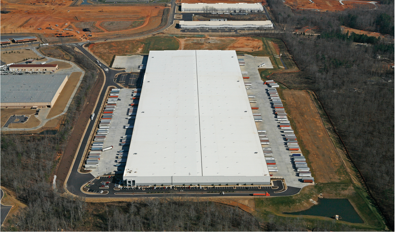
SouthPort Logistics Center
