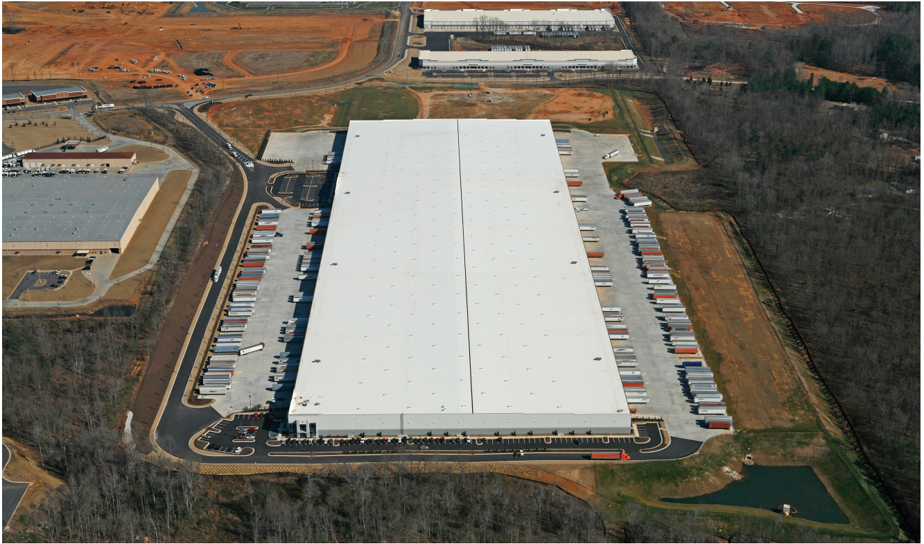
SouthPort Logistics Center
